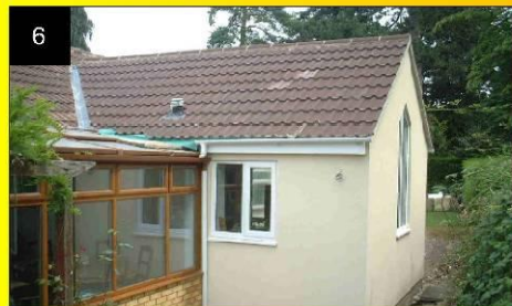
The completed kitchen extension.
