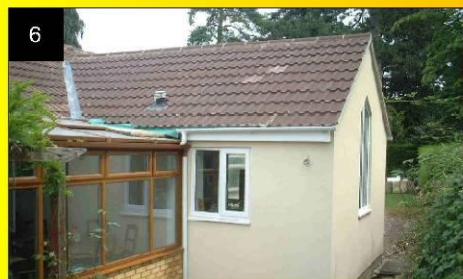
6 The completed kitchen extension.
