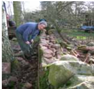
Wall maintenance by Pentalk member Jill Robson, from Ivegill
