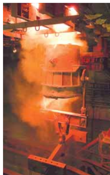
Right: Pouring of the Boat 4 Primary Shield Tank Top Casting at Sheffield Forgemasters in January 2007
