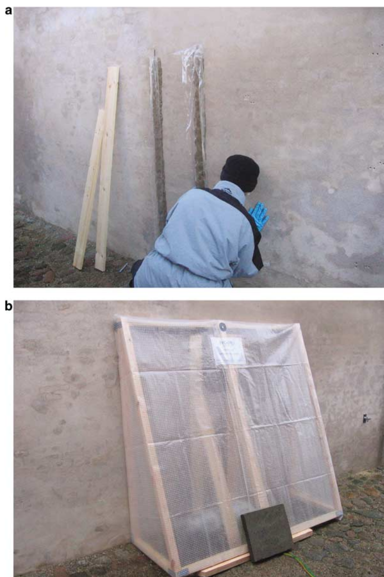
Figure 8: (a) The electrodes are placed at the masonry wall and (b) a tent protects the electrodes from rain and snow
