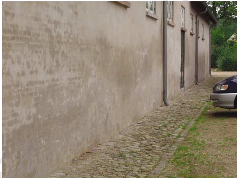
Figure 3: Hygroscopic moisture is seen as dark bands at a certain height
