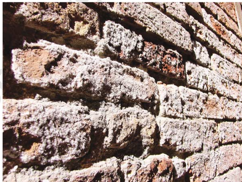
Figure 1: Salt-induced decay of brick masonry can be seen by the rounded corners. Salts have precipitated on the surface of the masonry as efflorescence
